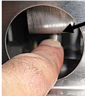
Filter Pump Reset Switch
